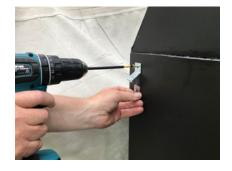
The large standoffs are for both the sides and the small ones go at the back. The small ones have to be screwed on each corner at the back of the firebox as shown in the image on the left.
